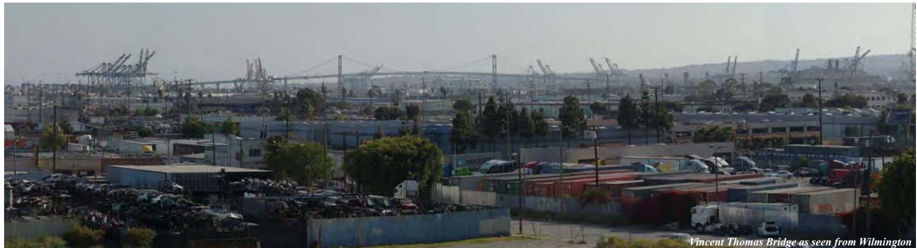
Vincent Thomas Bridge as seen from Wilmington
