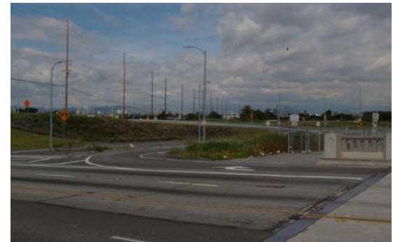
Challenging bike path entrance/exit at Lincoln Boulevard
