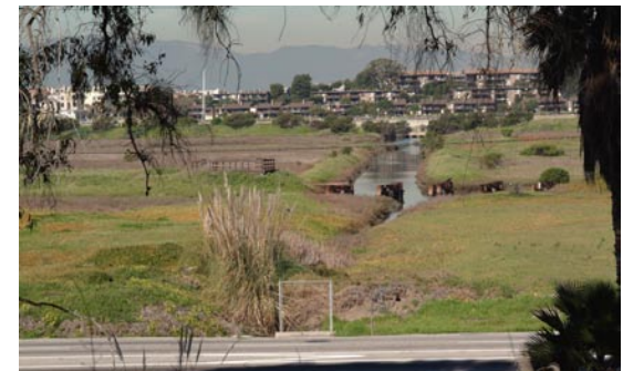
No fence at area B
