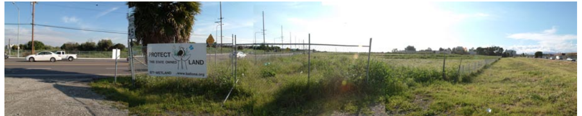
4. Culver Boulevard and Marina Expressway
