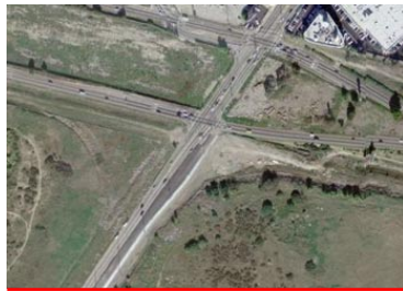
Culver Boulevard and Marina Expressway
