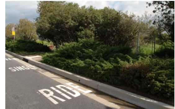
Existing bike lane at Fiji Way and location of proposed future Class I bike path
